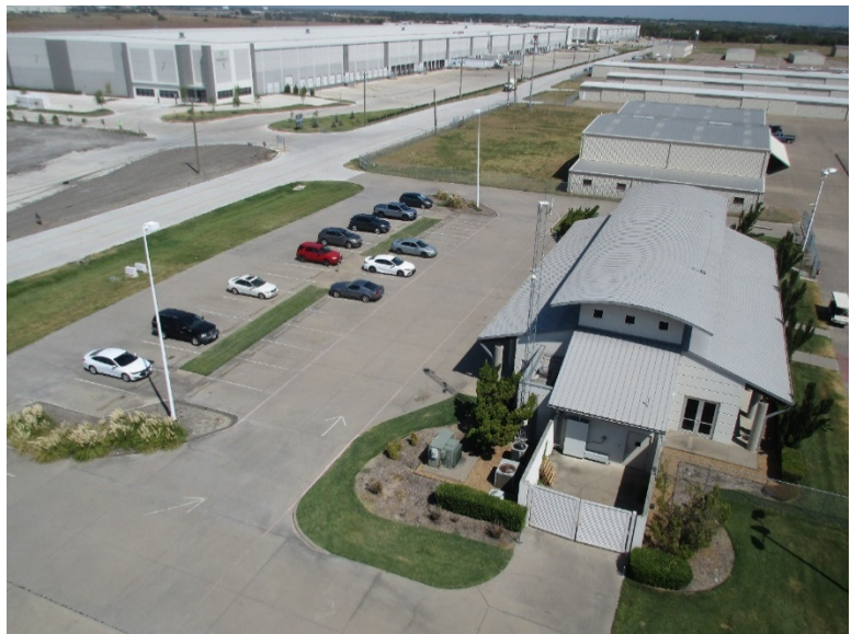
Terminal Parking Lot
