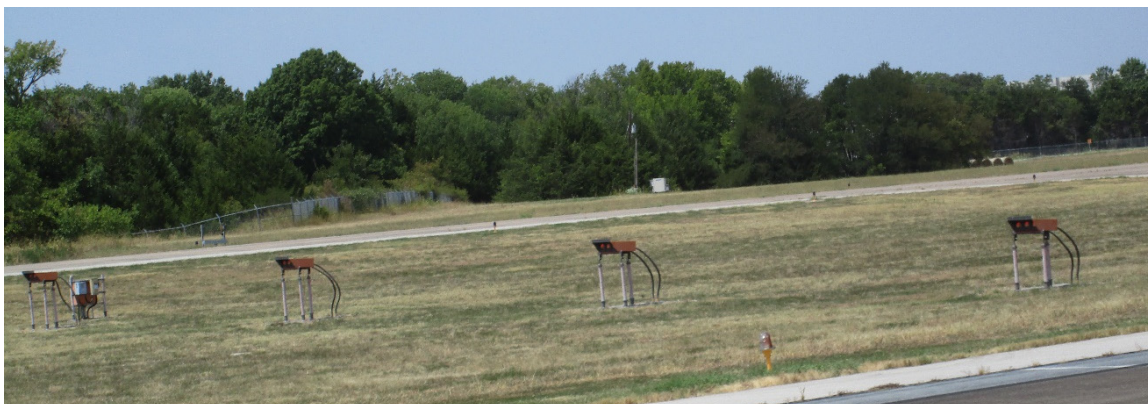
Precision Approach Path Indicator (PAPI) Visual Approach Lights
