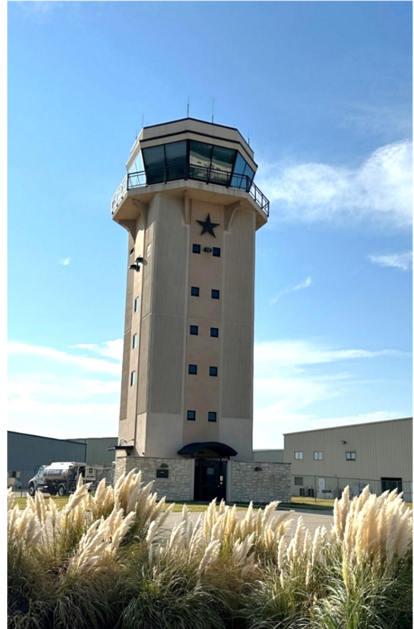
Airport Traffic Control Tower
