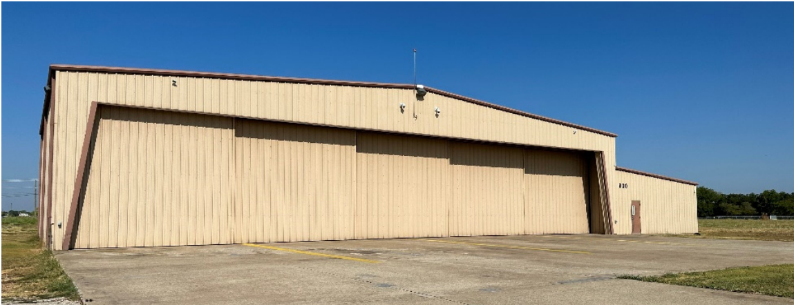
Executive Hangar - Building 900
